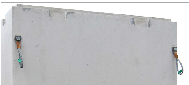
Four anchor straps facilitate transport handling and installation
